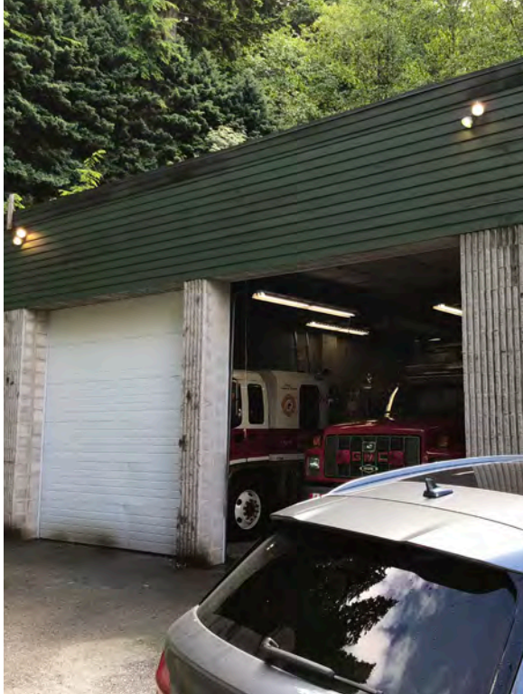
12' apparatus bay doors with less than adequate space for fire trucks.
