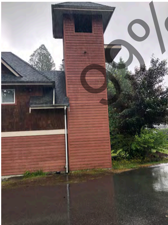
Training tower no longer usable for training, exterior wood panelling worn by elements.
