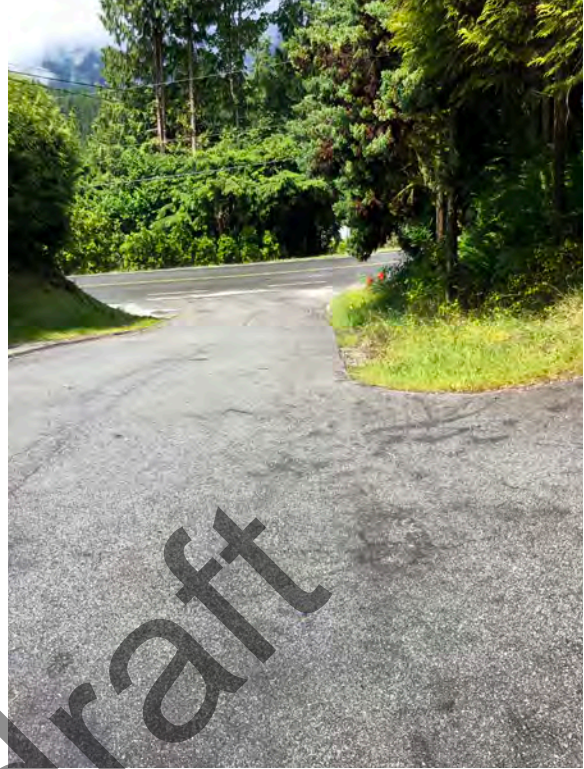
Sloped driveway with limited vision of traffic along Bedwell Bay Road - road approach at 8.3%
