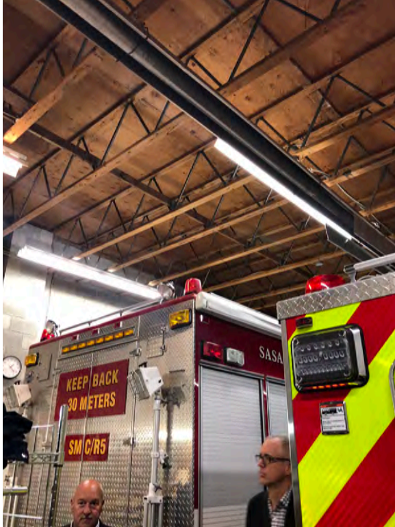
Exposed ceiling structure requires fire-rated enclosure.
