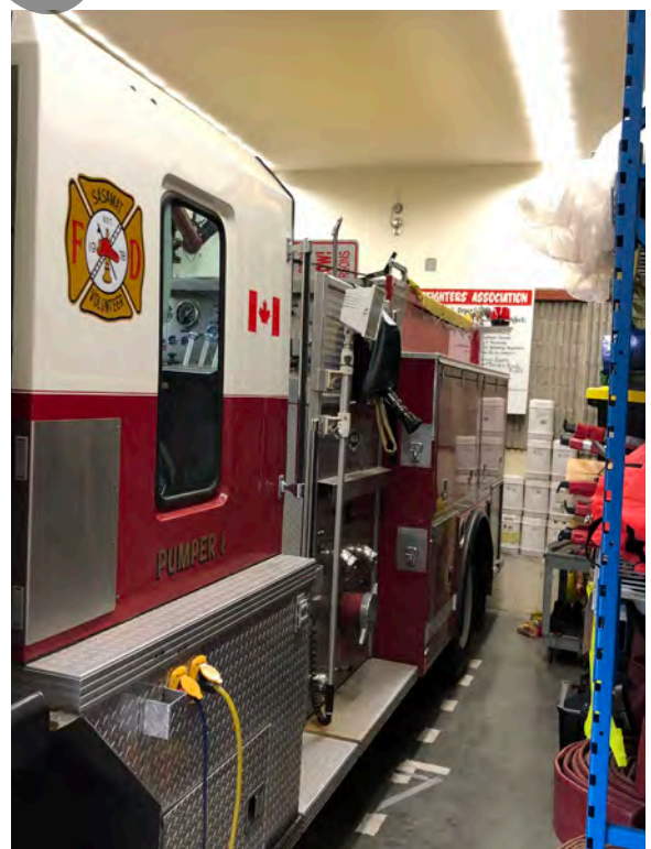
Circulation space around vehicles is inadequate and compromises personnel safety when trying to access vehicles quickly during an emergency
