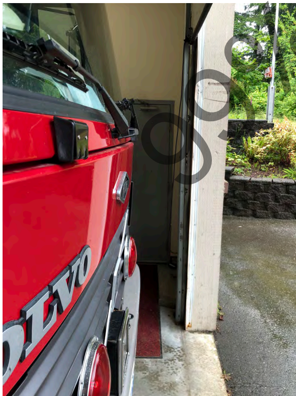
Less than 2 feet of space between apparatus and overhead door when closed.
