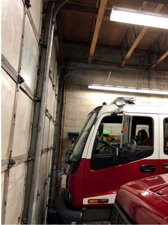
Extremely narrow space between truck and apparatus doors - limiting crew flow to gear & vehicles.
