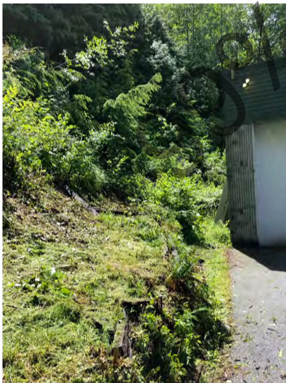
Firehall located against steep terrain with no retaining wall or slide protection.
