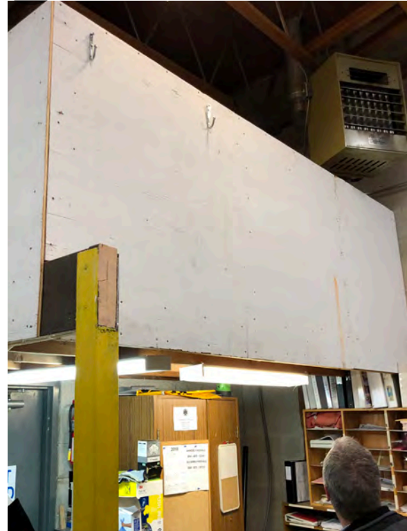
Makeshift storage located above filing area, not structural sound for post-disaster requirements.
