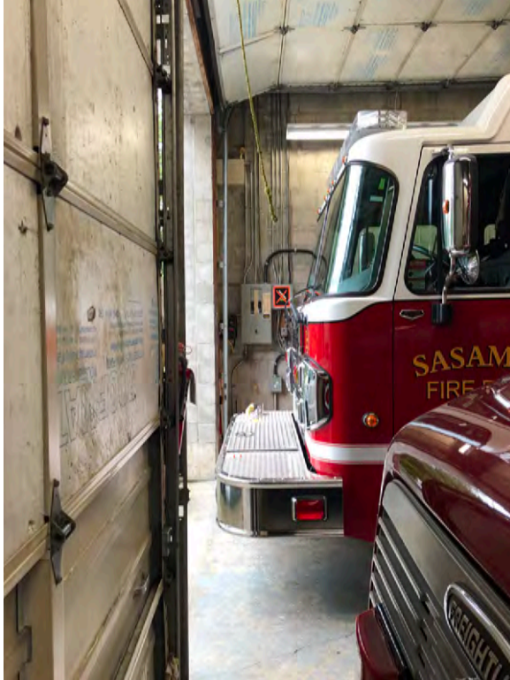
Apparatus bays with extremely limited space between vehicles and doors.
