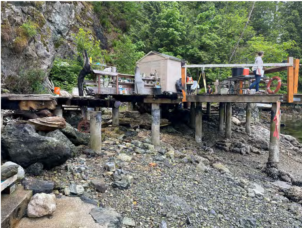
Photos from site inspection, May 31, 2022
