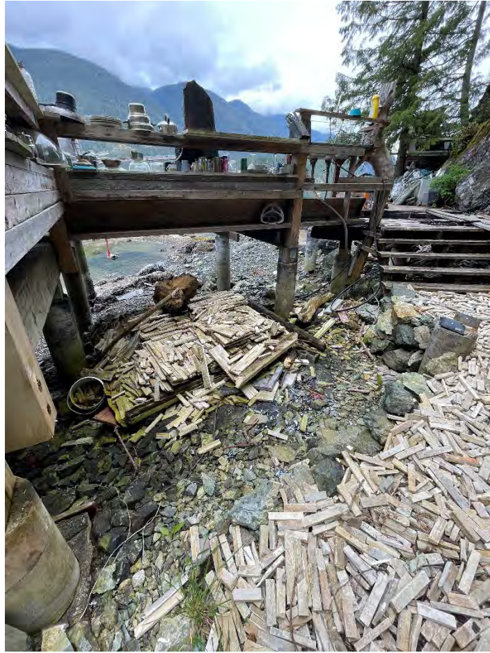
Photos from site inspection, May 31, 2022
