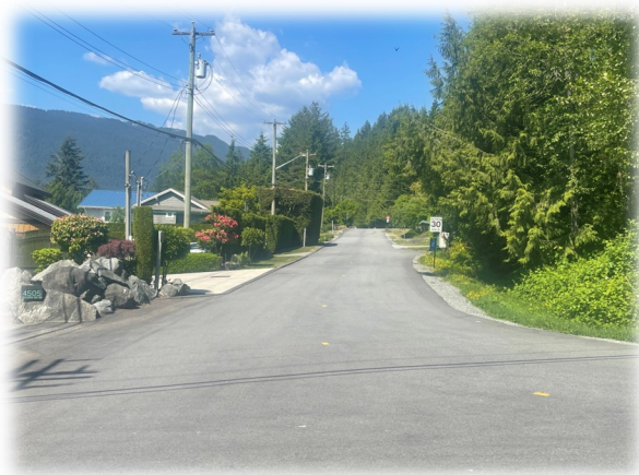
Belcarra Bay Road regrade and paving
