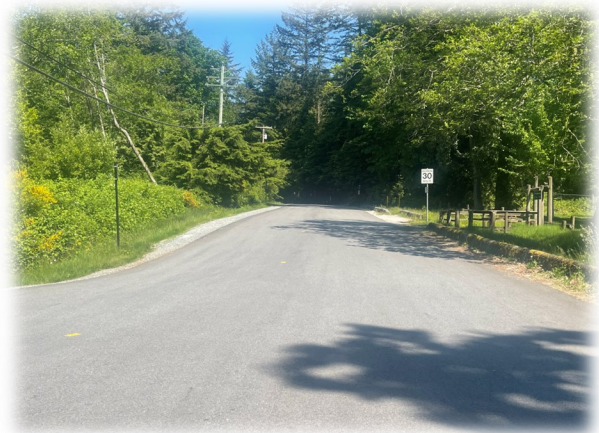
Midden Road regrade and paving
