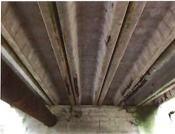
Figure 2.18 - Underside of original deck stringers looking south
