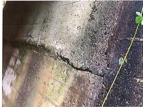
Figure 2.9 - Crack repair to northeast abutment
