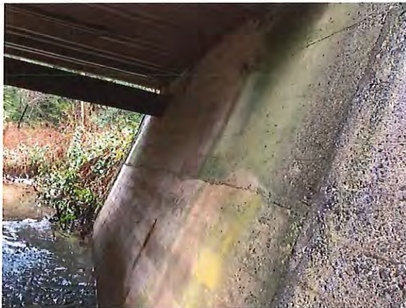
Figure 2.8 - Crack to south abutment
