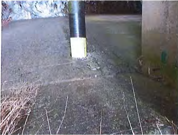
Figure 2.10 - Gas pipe connection at south abutment
