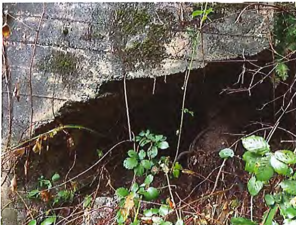
Figure 2.16 - Scour hole below northeast wingwall
