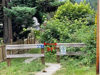
Perhaps 31" was regulation when the gate was installed, but now 1300mm = 51 inches is the minimum required gap. (from City of Coquitlam)
