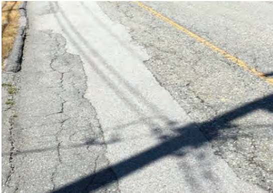
Level 2 Patch - In poor condition
