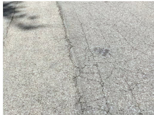
Inadequate crack sealing
