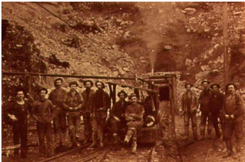
In those days jack hammers, operated by steam power, were already in use, and were used by crews of men in three eight-hour shifts, to drive a tunnel in two directions: one from the east and the other from the west. The broken rock was transported by a narrow railway system out of either end as the tunnels were only 9
