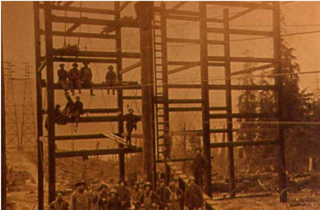
Hydroelectric transmission line construction from Buntzen power plant at Indian Arm to Greater Vancouver.
