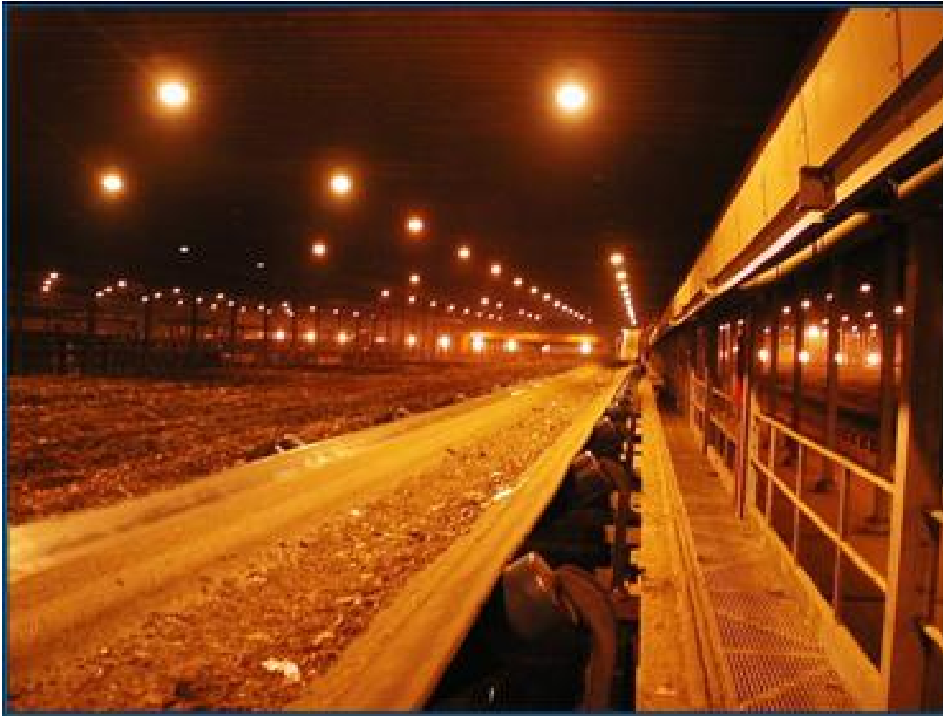
MBT Facility in Edmonton
