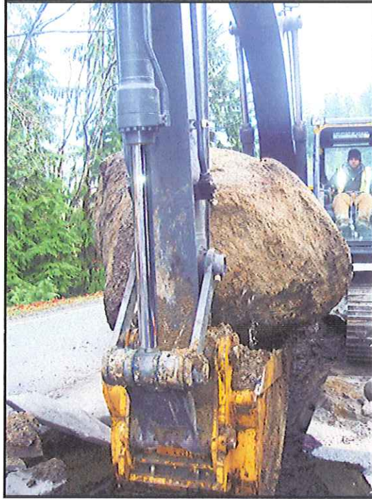
Photo 3 – Native material encountered under existing roads.
