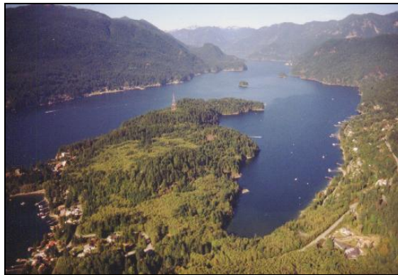
Figure 5: Bedwell Bay Looking North. Source: L. G. Scott, Sasamat Volunteer Fire Department .
