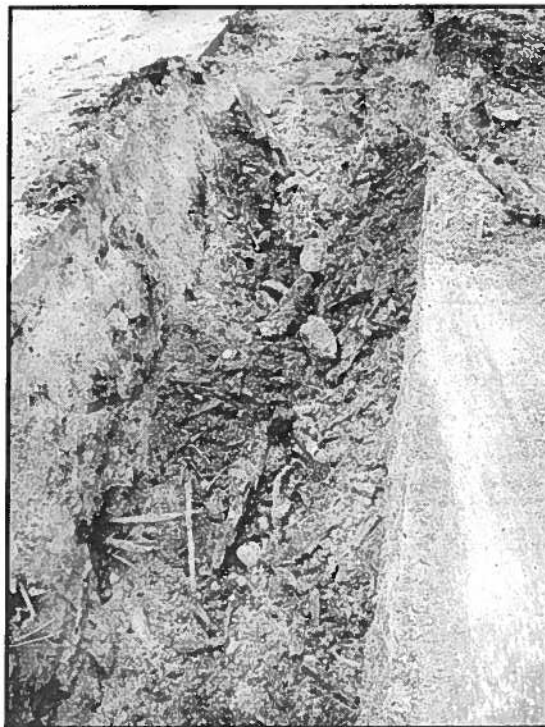
Photo 2 – Section of road constructed on woody organic debris
