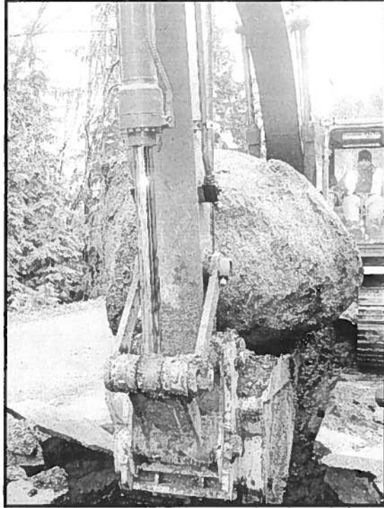
Photo 3 – Native material encountered under existing roads.
